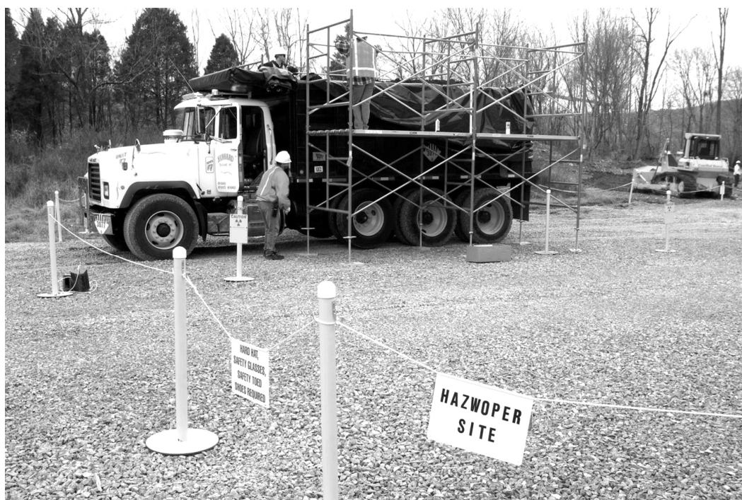
Fig. 3.8. Loading truck with waste for disposal.
