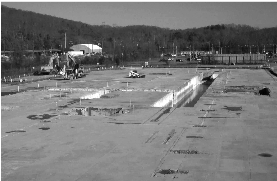
Fig. 3.6. K-1420 footprint after demolition.
