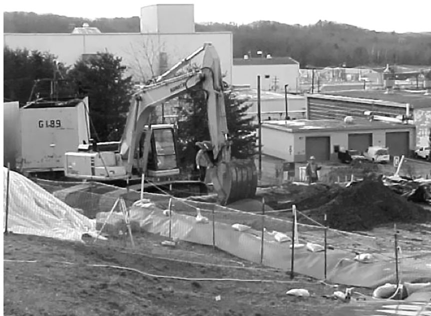
Fig. 3.7. Remediation of soil at East Tennessee Technology Park.
