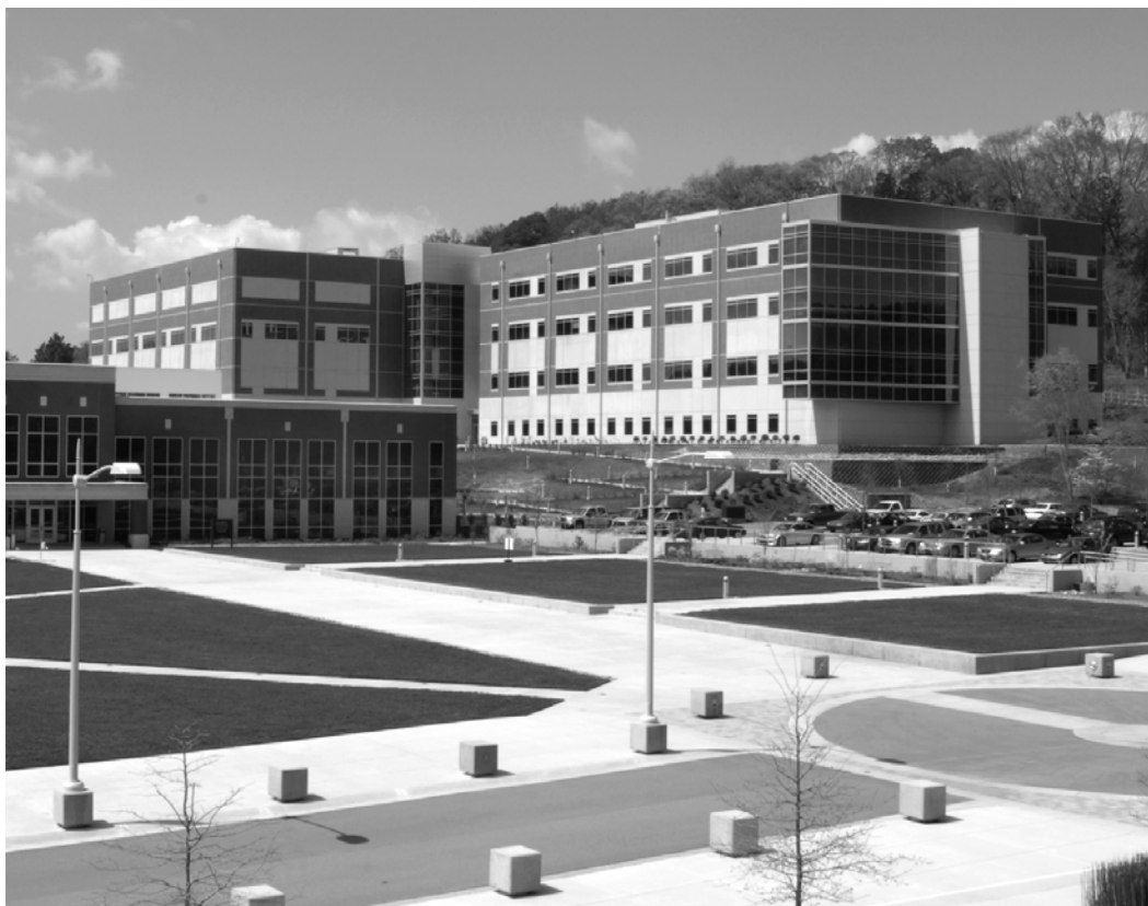
Fig. 5.2. The Oak Ridge National Laboratory Multiprogram Research Facility—Leadership in Energy and Environmental Design (LEED) Gold.
