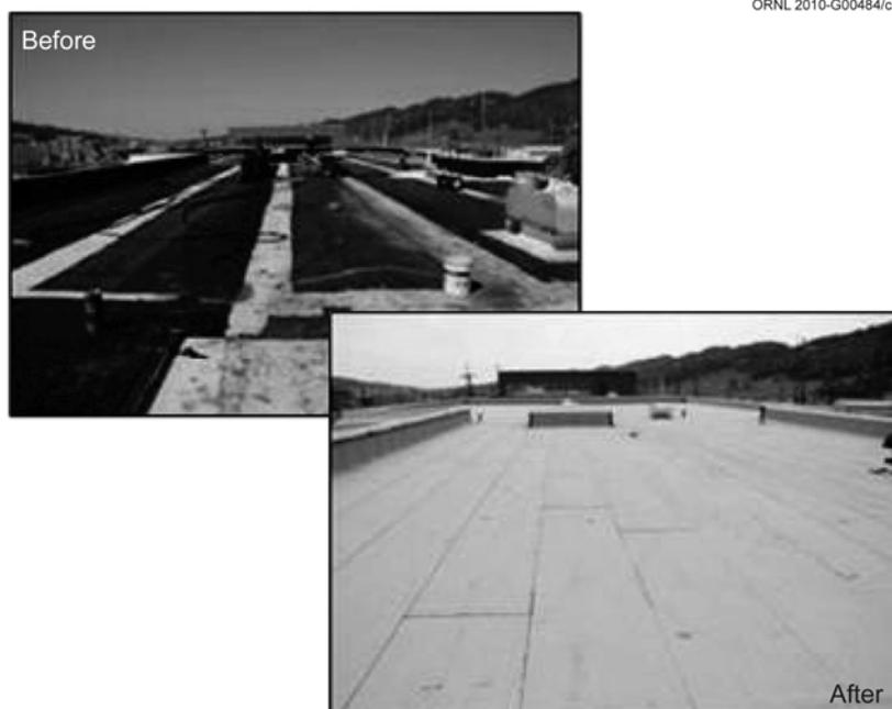
**Fig. 4.12. Replacement of deteriorated roof on Building 9113 with a sustainable white roof.**
