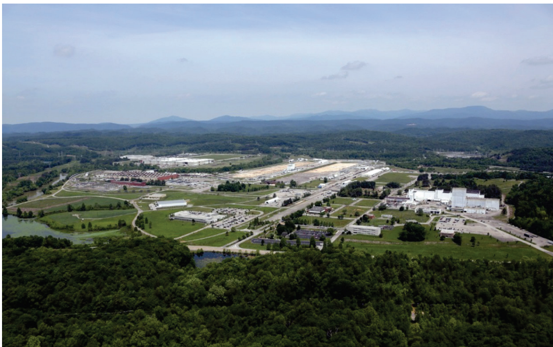
Fig. 1.8. East Tennessee Technology Park.
