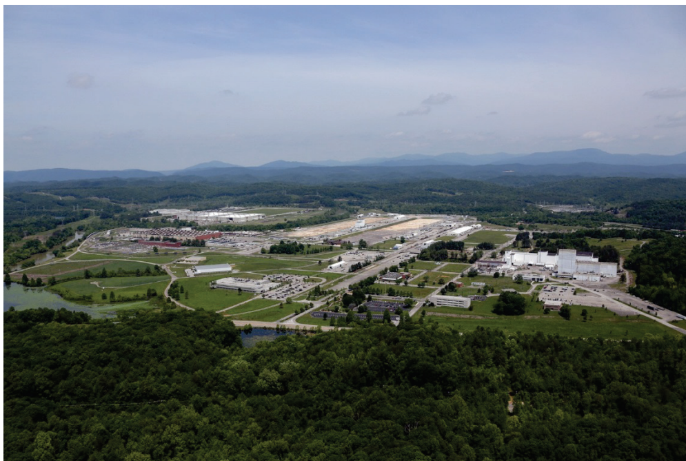
Fig. 3.1. East Tennessee Technology Park.
