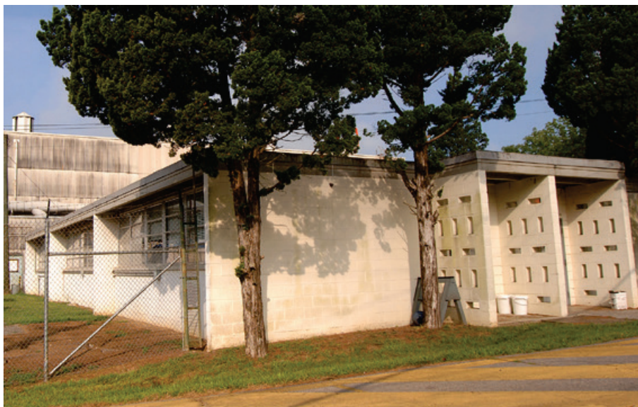
Fig. 5.40. Molten Salt Reactor Experiment Facility.
