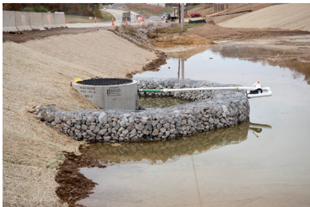
Fig. 4.13. Faircloth skimmer previously installed at Sediment Basin 1.
