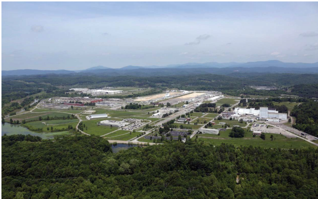
Fig. 1.8. East Tennessee Technology Park.
