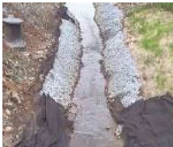
Figure 3.44. Construction of lined section of Mitchell Branch, MIK 0.7, in 1998
