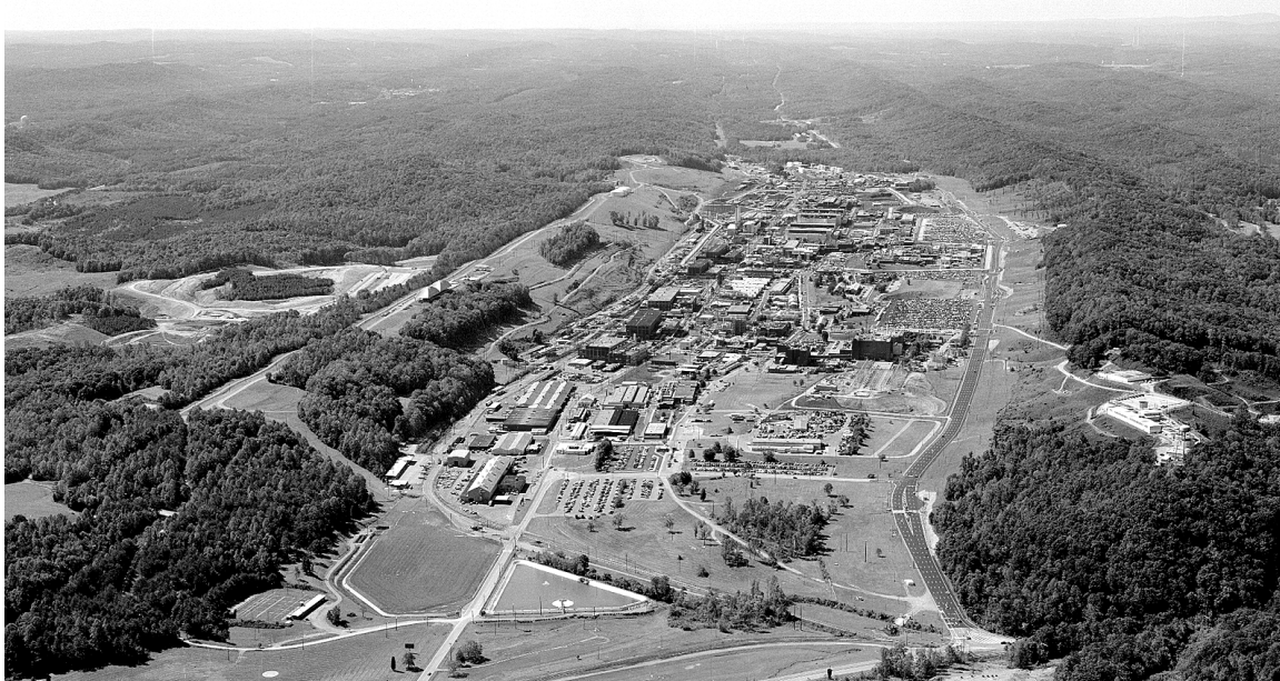
Fig. 1.8. The Y-12 National Security Complex.
