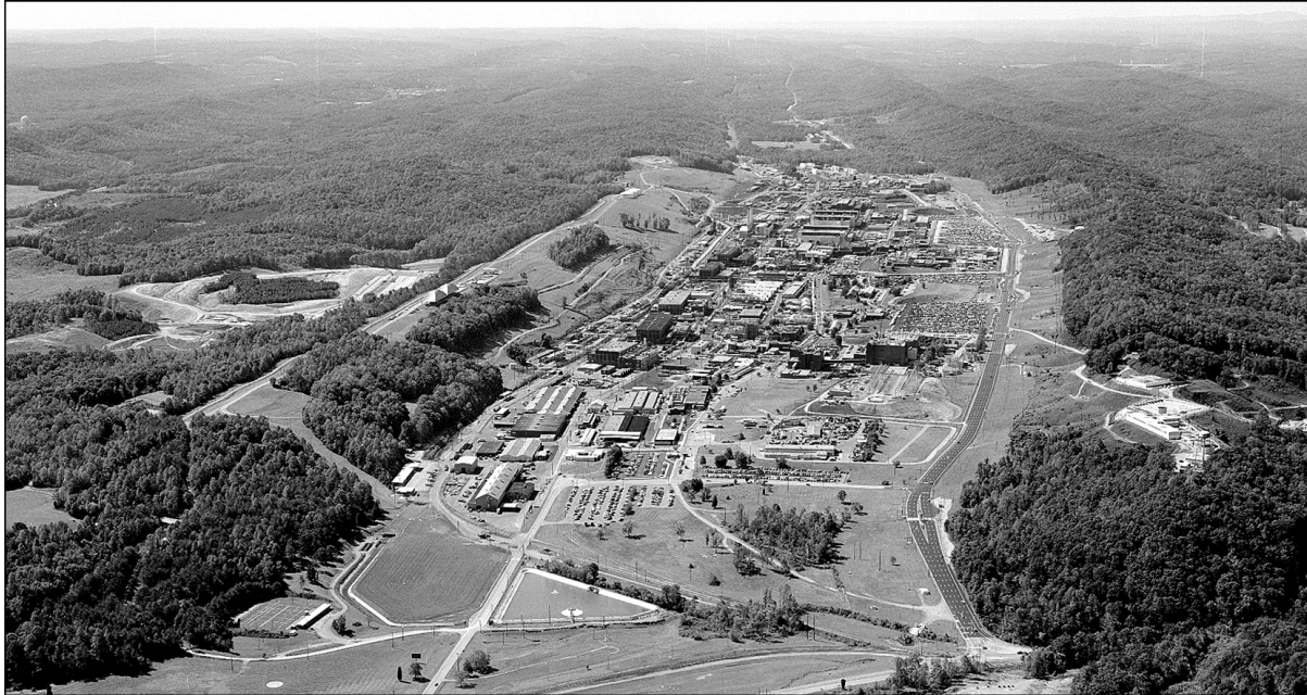
Fig. 1.8. The Y-12 National Security Complex.
