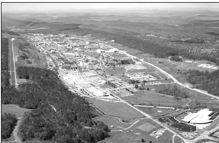
Fig. 1.7. Y-12 National Security Complex.
