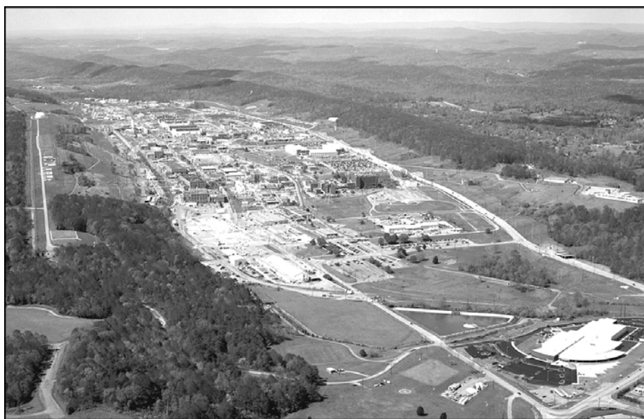
Fig. 1.8. Y-12 National Security Complex.
