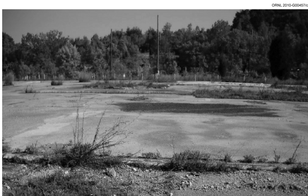
Fig. 3.18. The K-1420 pad after demolition.
