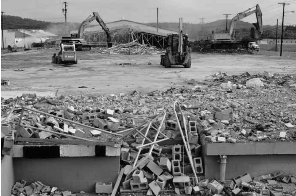
Fig. 3.23. K-1035 building demolition.
