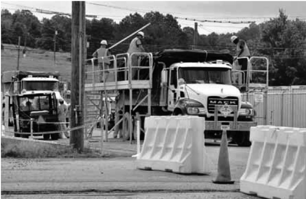
Fig. 3.24. Demolition debris generated from K-1035 building being sent to EMWMF.
