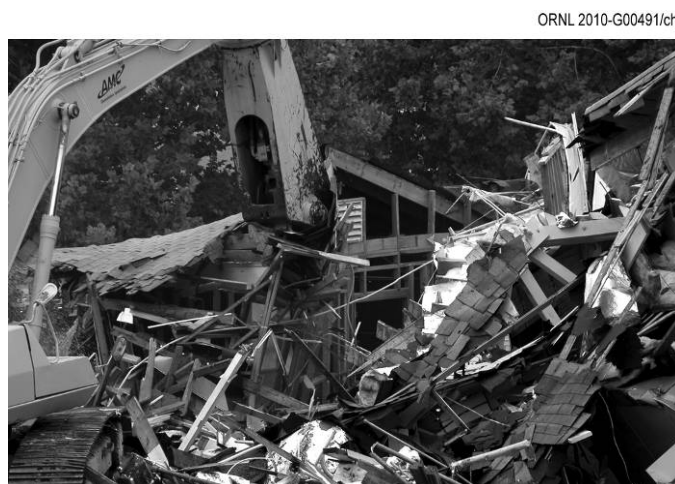
Fig. 5.6. Demolition activities at ORNL.
