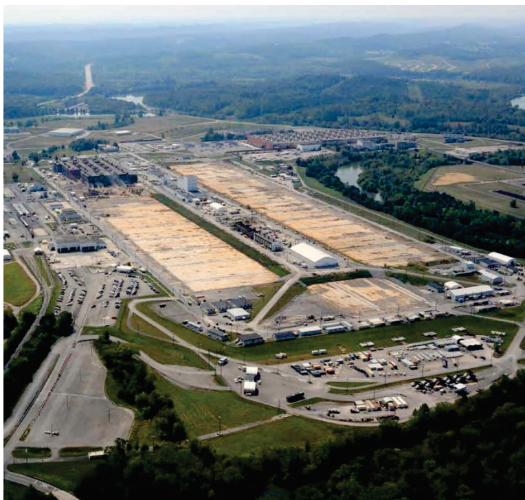
Fig. 3.57. Building K-25 in late 2013.
