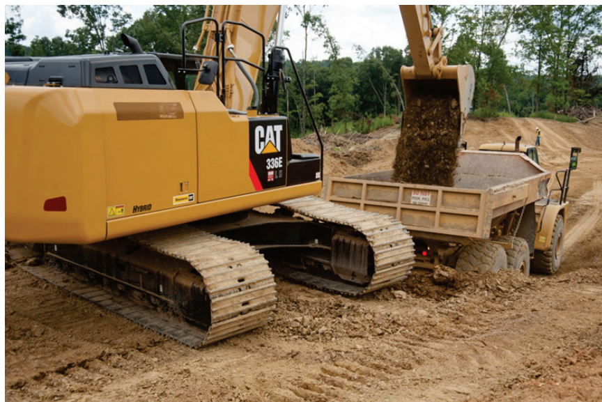
Fig. 4.11. Hybrid excavator used for Uranium Processing Facility site preparation.
