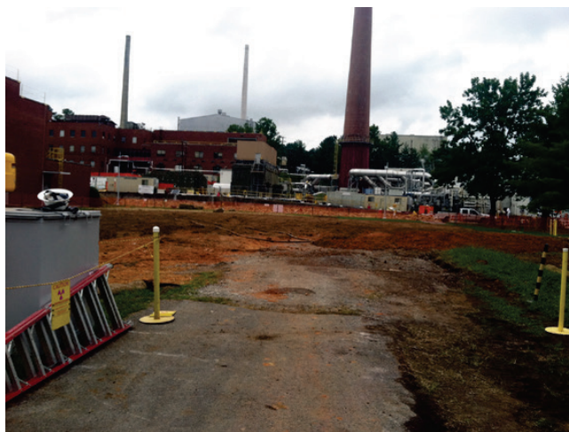
Fig. 5.41. Building 3550 area after being cleared.
