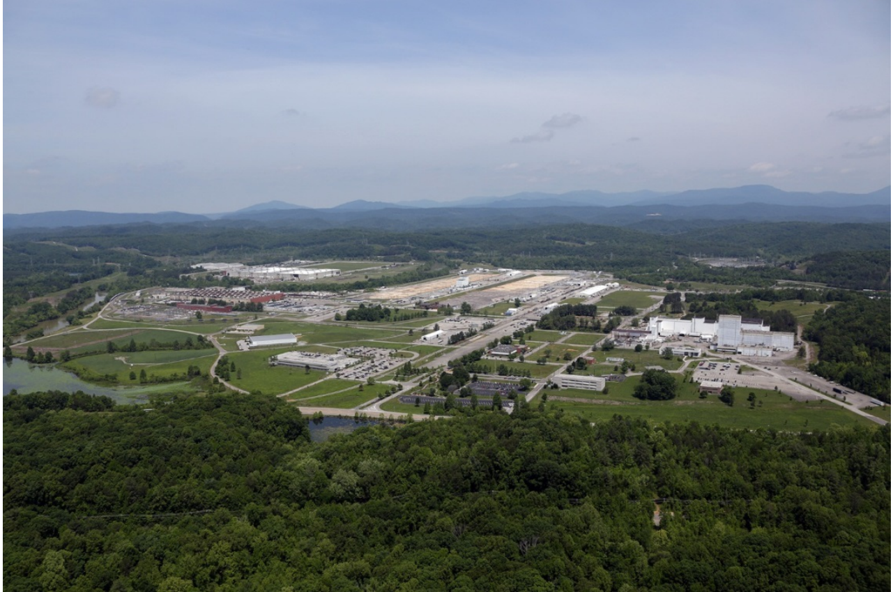
Fig. 3.1. East Tennessee Technology Park.
