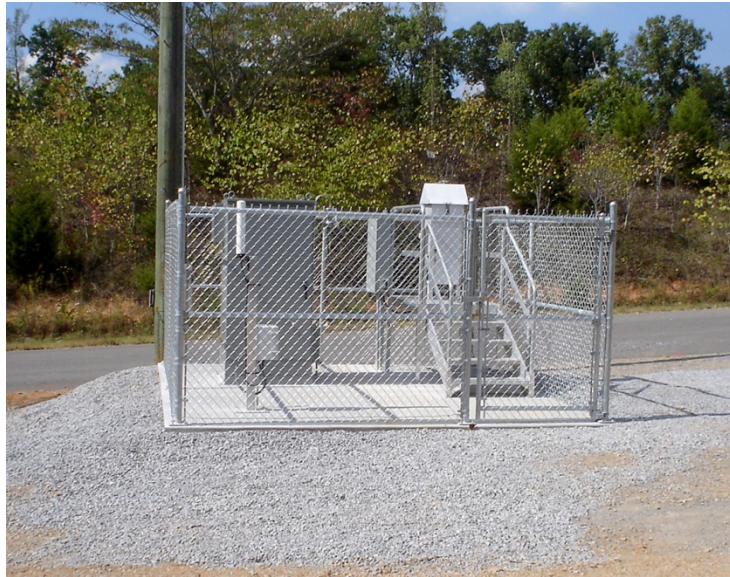
Fig. 6.3. Oak Ridge Reservation ambient air station.
