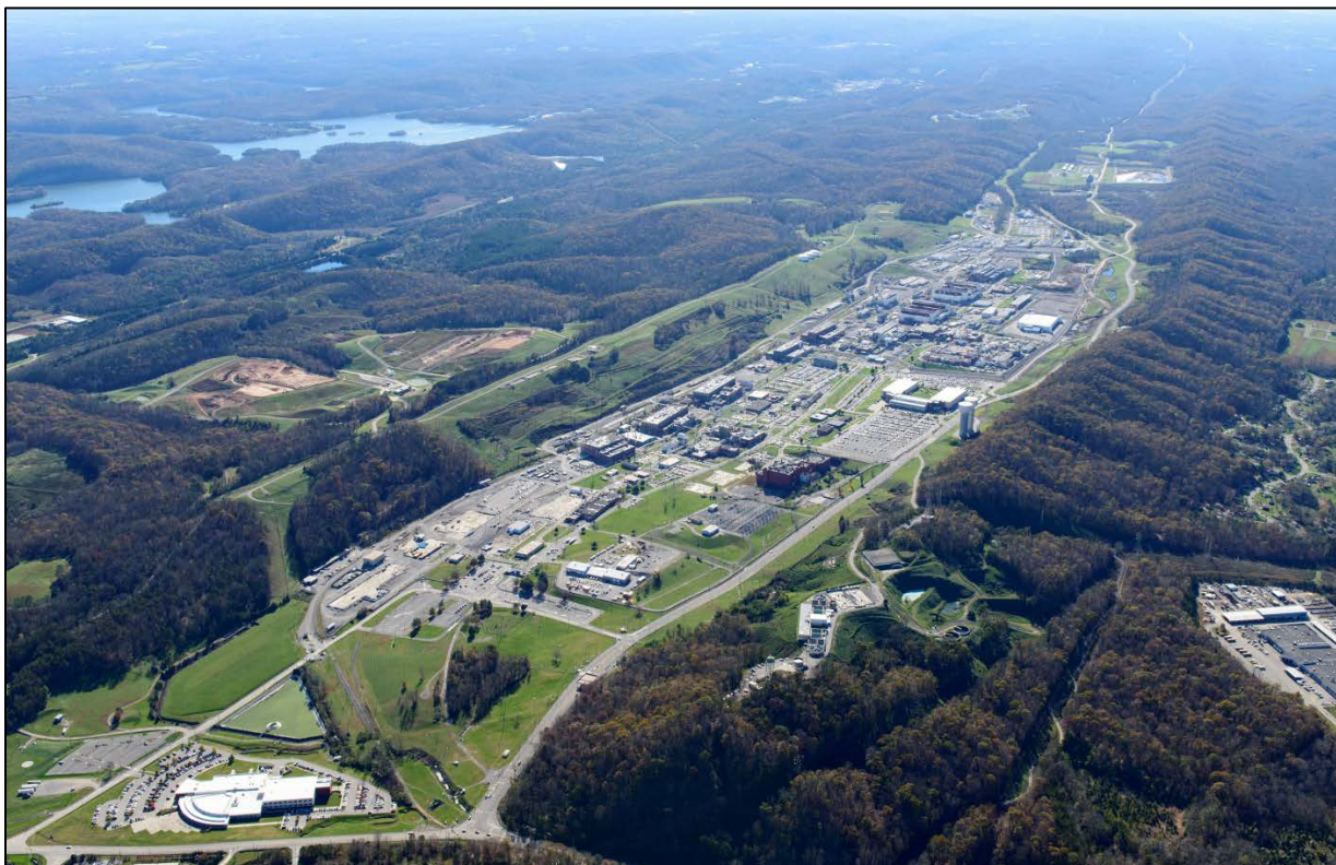
Figure 1.7. Aerial view of the Y-12 National Security Complex
