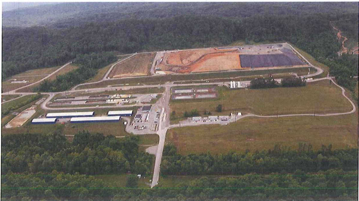
Figure 2. Environmental Management Waste Management Facility.
