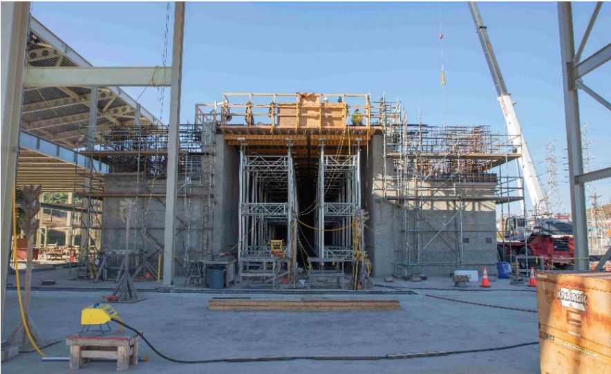
Figure 8. Treatment Site - south side looking west. Treatment Filter building under construction, with second-level concrete slab held up with shoring.
