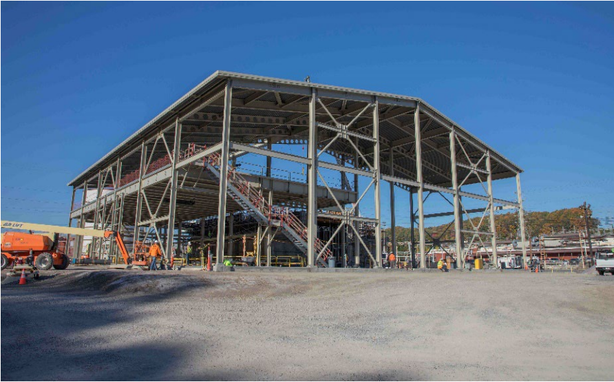
Figure 6. Treatment Site - southeast side looking west. Treatment building under construction.
