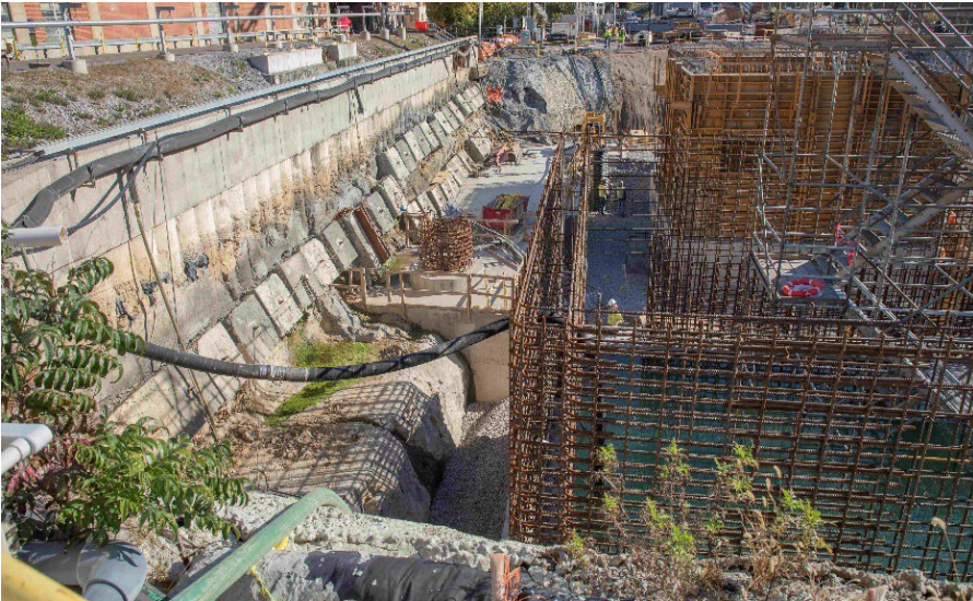
Figure 4. Headworks Site - west side looking east. Storm Flow Pump Station in foreground, Grit Pump building behind. Secant wall and anchoring system on left.
