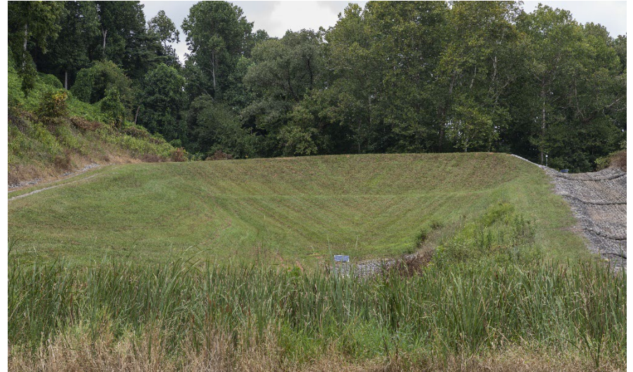
Figure 6. FCAP berm and spillway.
