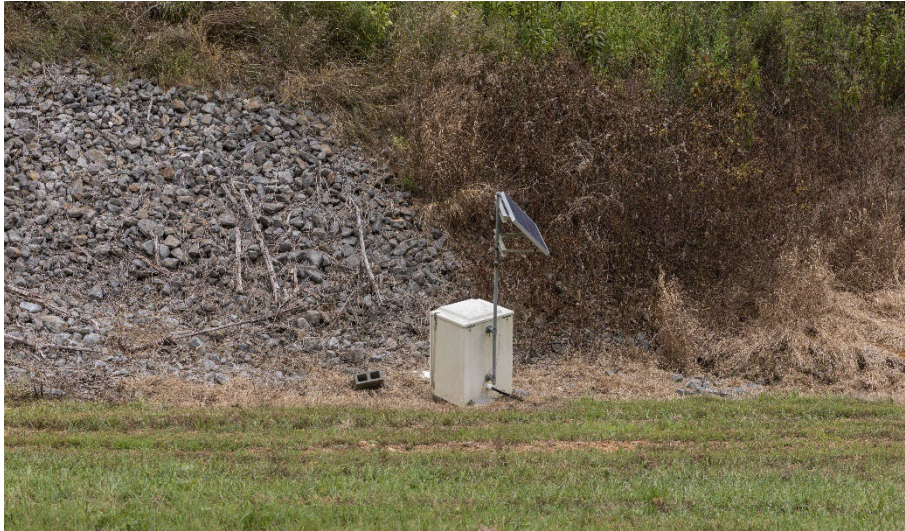
Figure 5. Leachate influent monitoring station (MCK 2.05) at head of passive treatment wetland.
