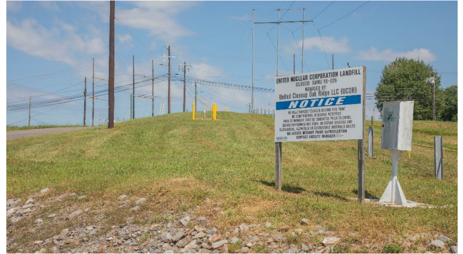
Figure 4. UNC Disposal Site (looking east/southeast) with monitoring well in background.
