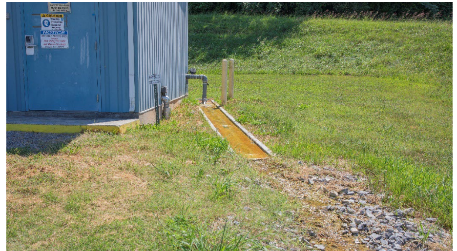
Figure 4. Concrete swale constructed in March 2023 to bypass the underground discharge piping.
