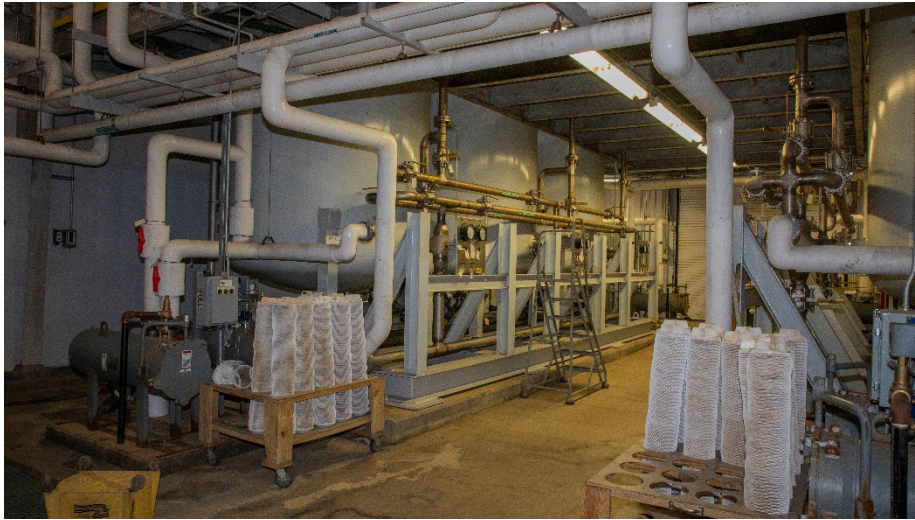
Figure 1. Activated carbon column bank with particulate pre-filter on lower left.
