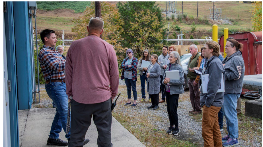
Figure 8. BSWTS facility manager (left) explains treatment system operations to 2024 FYR site visit participants.
