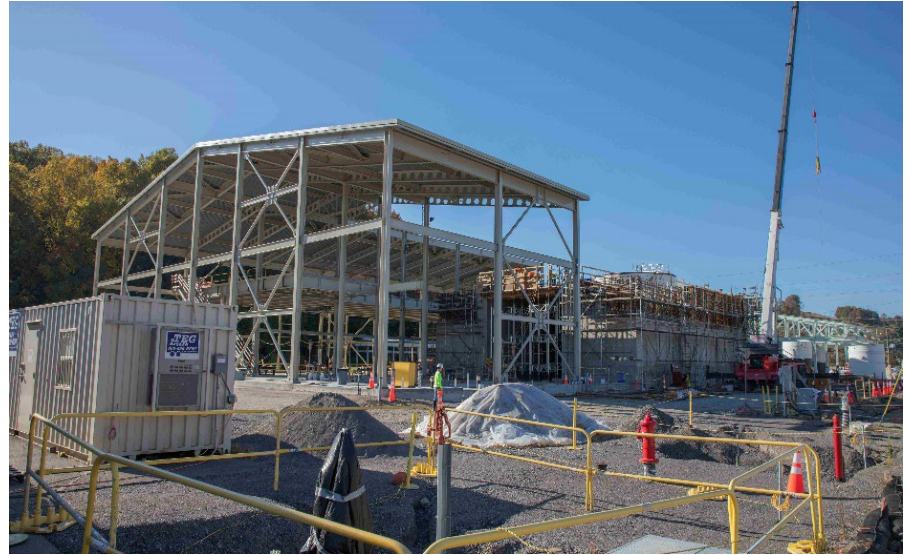
Figure 7. Treatment Site - northeast side looking west. Treatment building under construction (center), chemical storage tanks on right.
