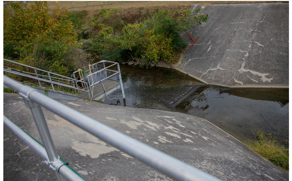
Figure 6. UEFPC Station 17 IP surface water sampling station.
