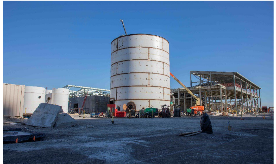
Figure 9. Treatment Site - south side looking east. Chemical reaction tanks awaiting placement (left). Equalization tank (center) and treatment building (right) under construction.
