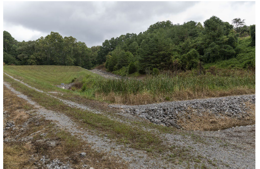
Figure 8. FCAP in background with the passive wetland and access roads in the foreground.
