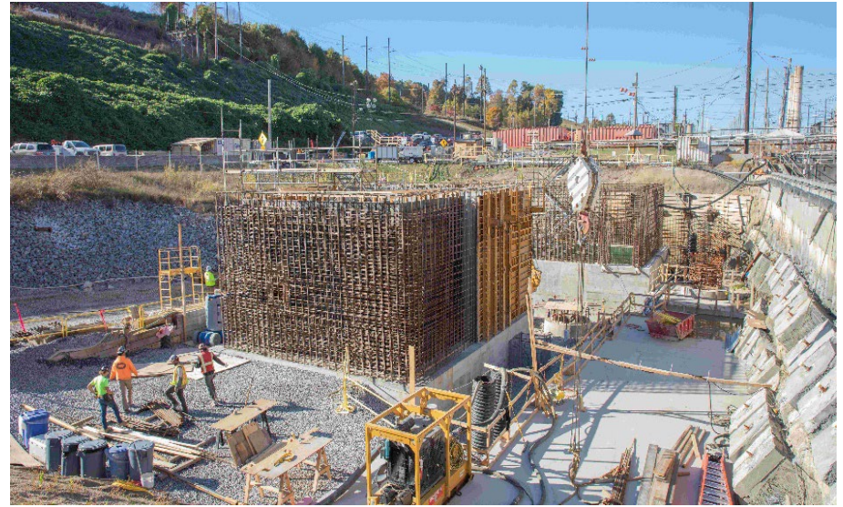
Figure 3. Headworks Site - east side looking west. Grit Pump building (center) and Storm Flow Pump Station (right) under construction.
