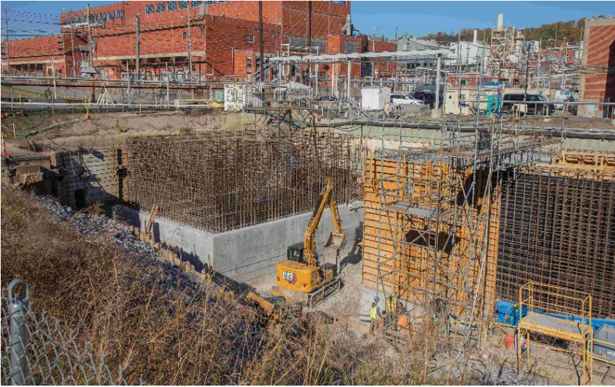
Figure 2. Headworks Site - south side looking northwest. Storm Flow Pump Station (left side) and Grit Pump building (right side) under construction.
