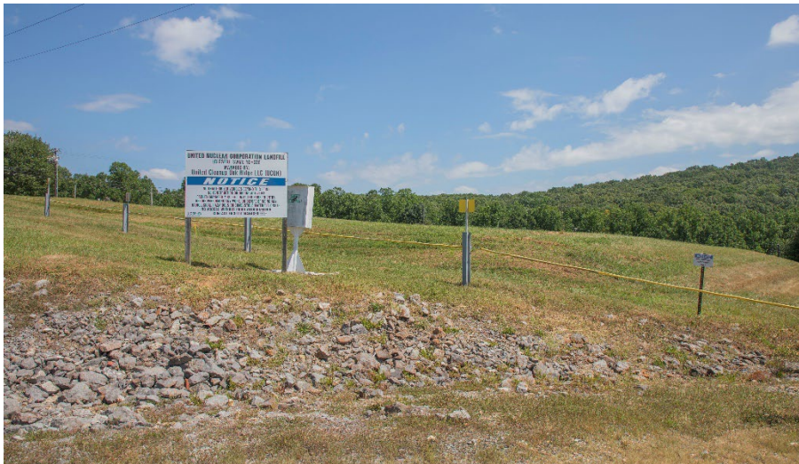
Figure 3. View of UNC Disposal Site on ChR; note riprap around the perimeter of the site to control drainage (looking east).
