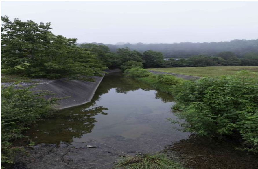
Figure 7. UEFPC concrete-lined channel viewed from LRBP-1.
