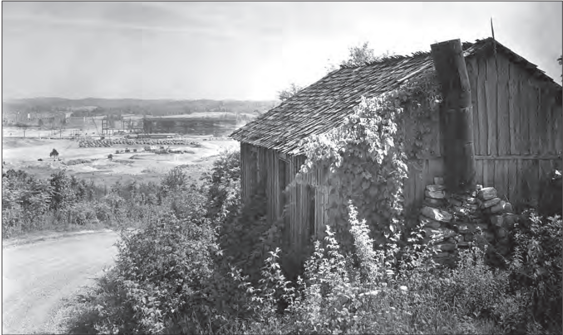
A. Original Farmhouse with K-25 under Construction, 1942
