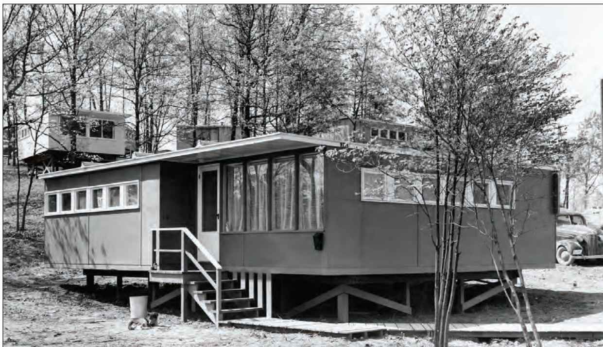
B. Prefabricated Flat Top Working Housing
