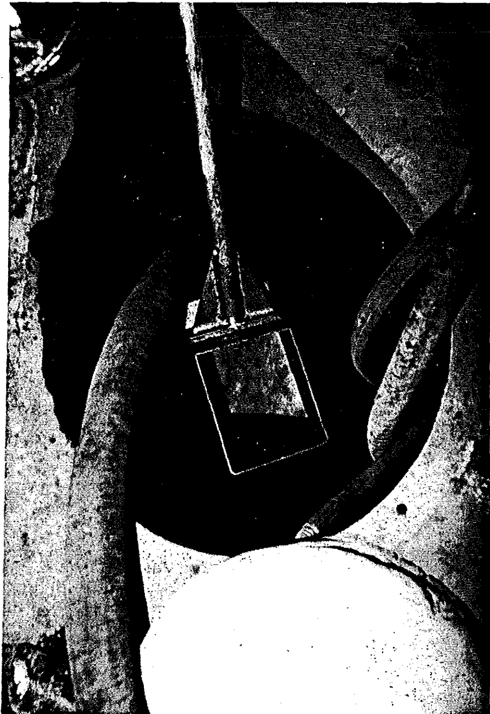
Fig. 3.4. Basement sump containing 6,000 lb of mercury in Building 9201-4. (1983 photo)
