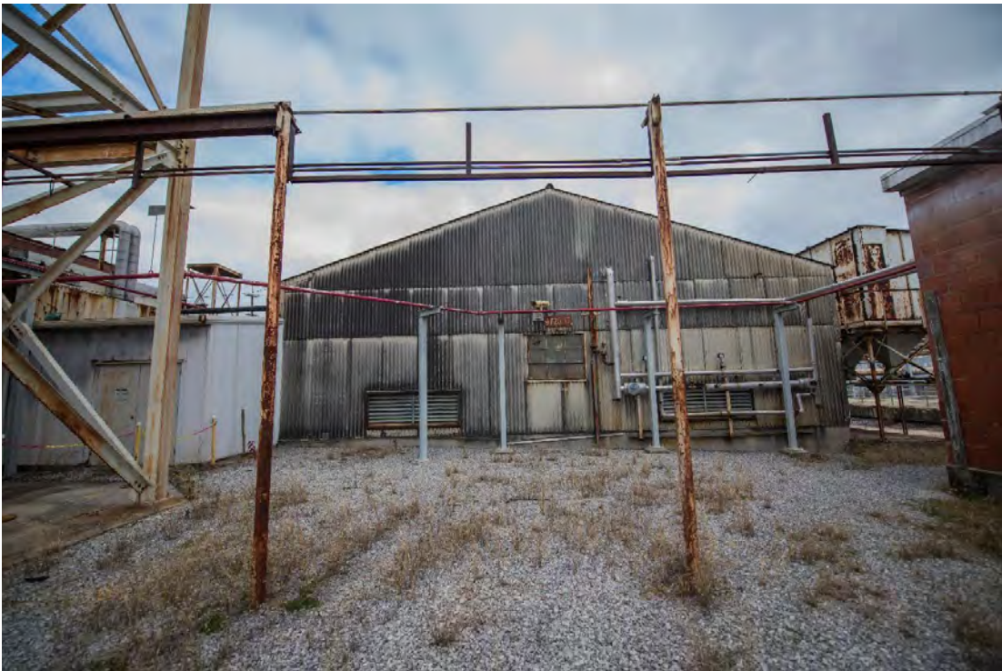
View of west side of building looking east
