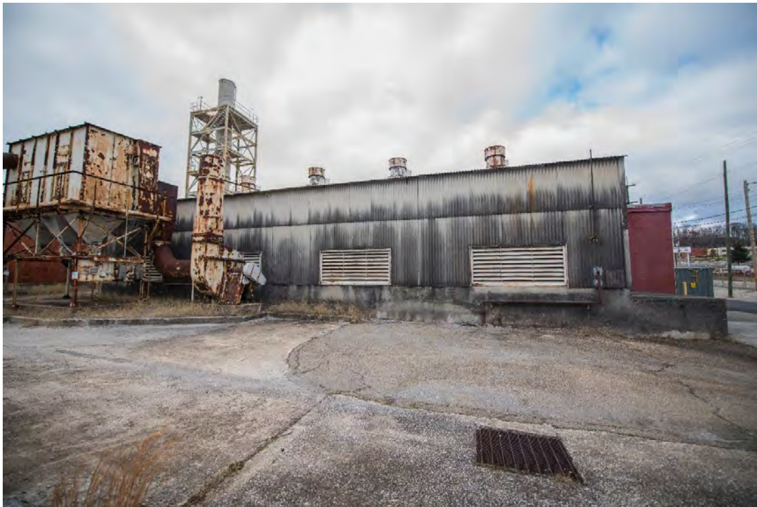
View of south side of building looking north
