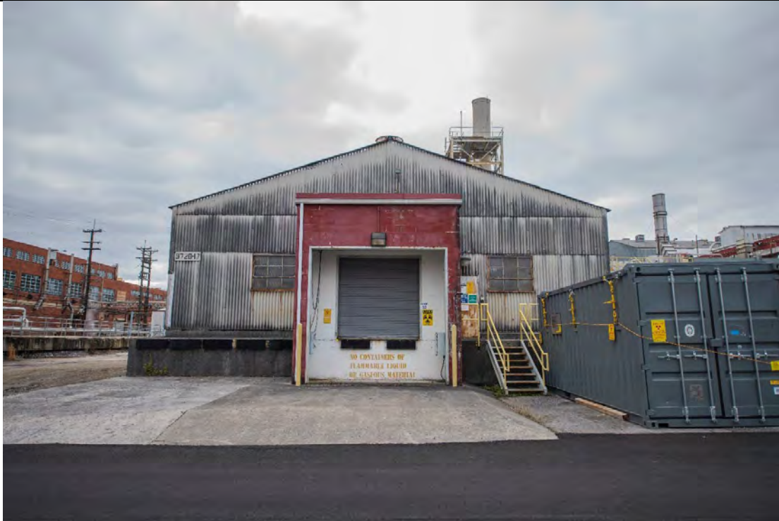
View of east side of building looking west
