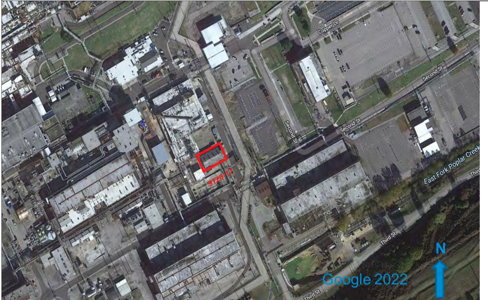
Figure 2. Aerial View of Building 9720-17
