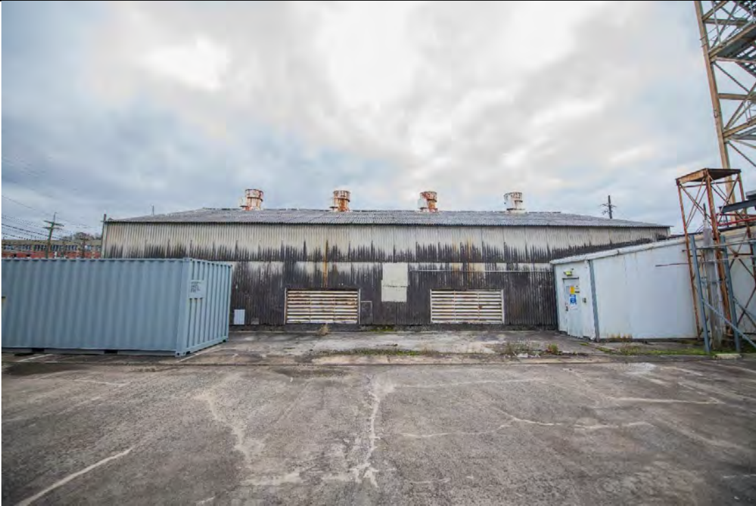
View of north side of building looking south
