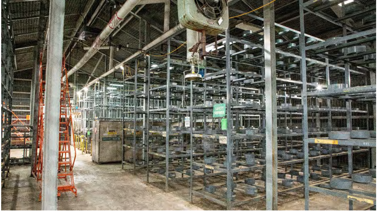
Figure 4. HEU storage racks (YPH-24-1150967)
