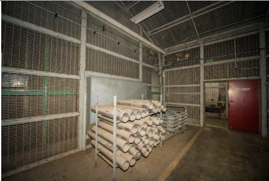
Figure 6. Photo of Building 9720-17 Interior
