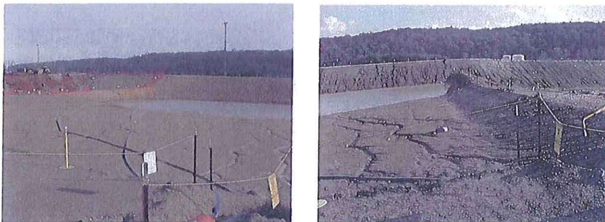
Figure 4: Flooded Cell 2 and repaired EMWMF berms.
