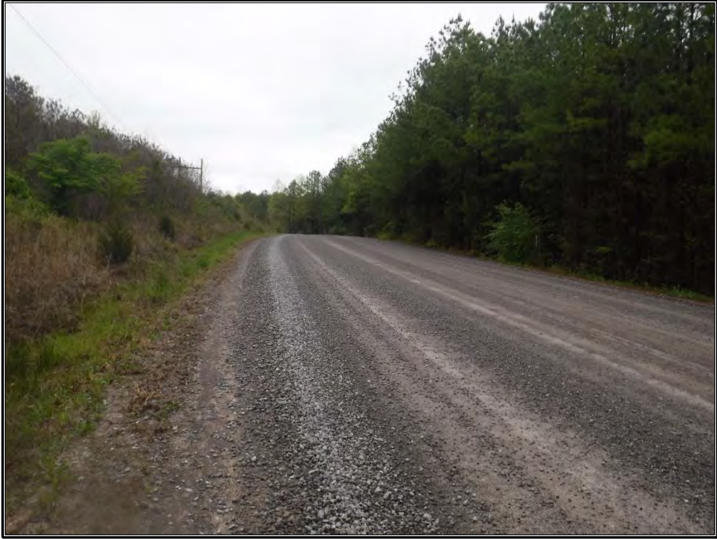
Figure 6. Overview of Haul Road, facing east.
